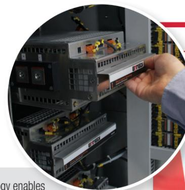
Removable module technology enables production to continue at a reduced speed in the event that a module fails. Take advantage of our *regional module exchange program* to exchange your module at one of our vast global service centers.
